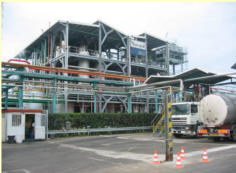
Figure 21: Biodiesel plant in Livorno, Italy
