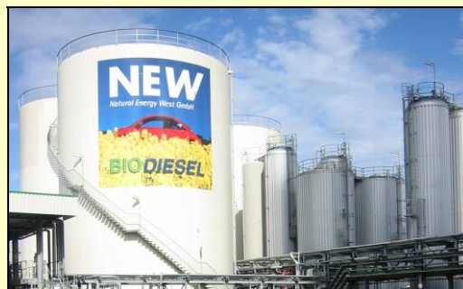
Figure 30: Tank farm of the NEW biodiesel production plant
