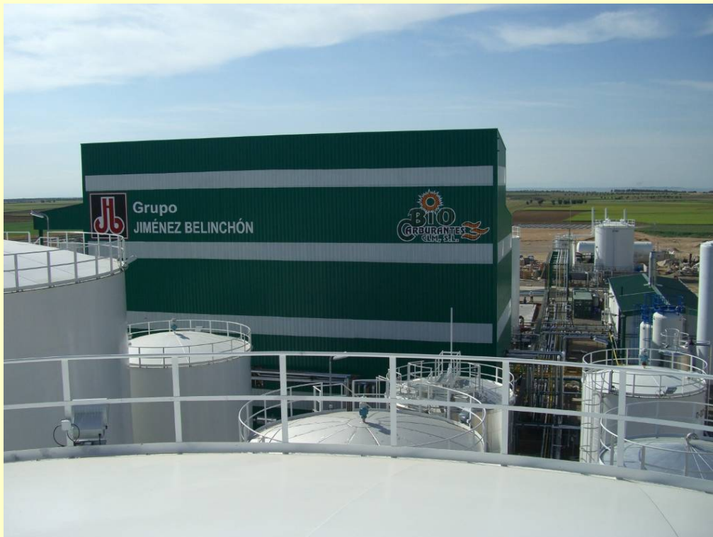
Figure 16: Production Facility in Ocana, Spain
