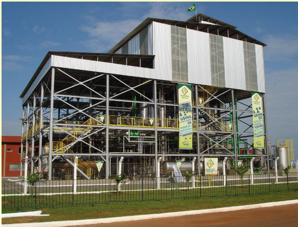
Figure 24: View of the biodiesel plant in Barro do Bugres, Brazil
