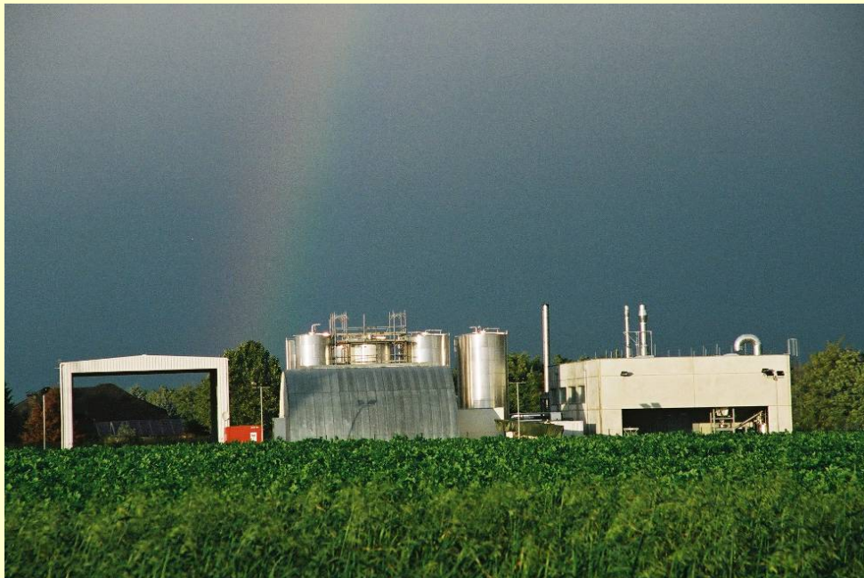
Figure 26: Delivery Unit, Tank Farm, Processing Unit
