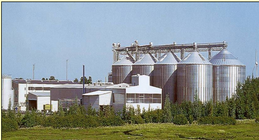
Figure 18: General view of the oil mill and Biodiesel plant in Falkenhagen
